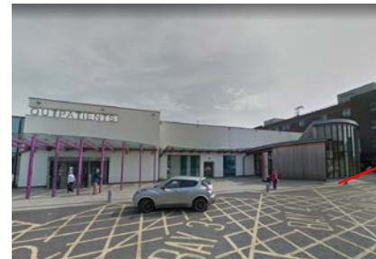
South Tyneside District Hospital
